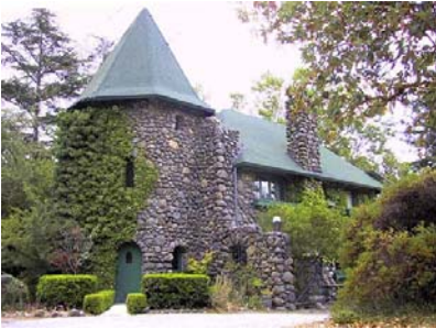
Gate House, Willowbrook
