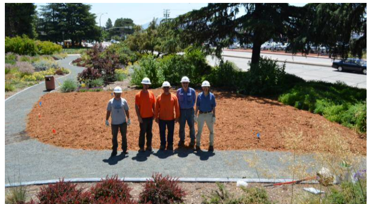
Sheet Mulching Completed
